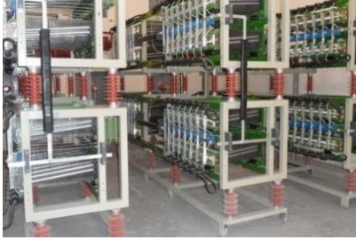
Installing SVC In Industrial Facilities
